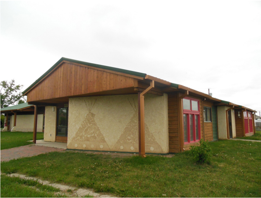
Cuts Wood School, Browning, Montana Photo by Mizuki Miyashita, 2014
