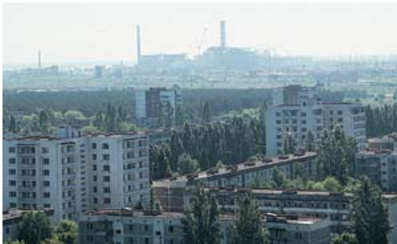
Figure 3. Pripyat, now abandoned, lies a mere 3 kilometers from the Chernobyl Nuclear Complex, which is visible on the horizon. Brenda Rodgers of Texas Tech University and author Chesser measured the radiation levels of every building in Pripjat, and the city is now the basis of a digital, three-dimensional reconstruction that models the flow of radiation in urban environments. (Photograph courtesy of the authors.)
